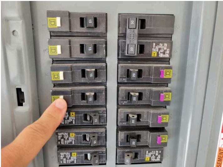
AFCI breakers checked
