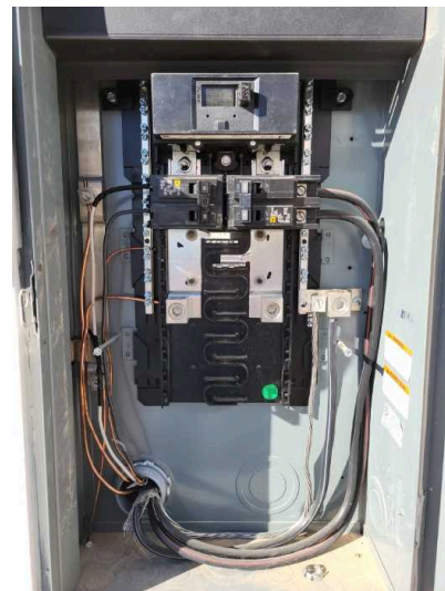
Electrical Main Cut Off
