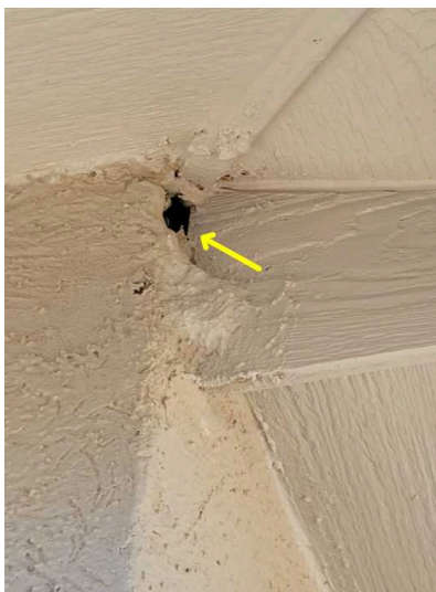
Seal the area where the wall and the soffit meet
