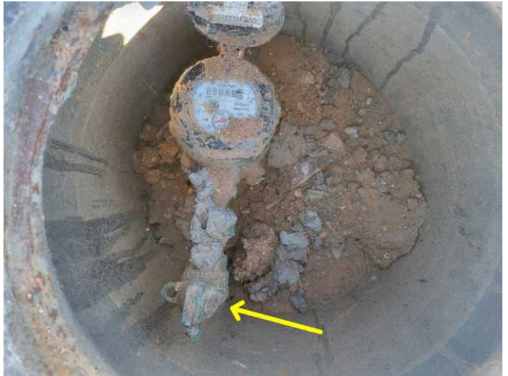
Water cut off is near the street
