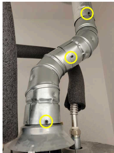
Drywall screws are not approved for the flue pipe and sheet metal.
