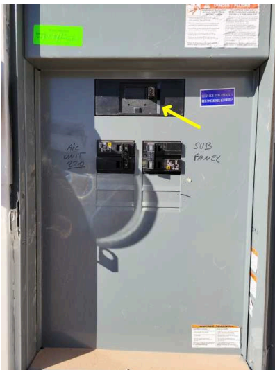
Electrical Main Cut Off
